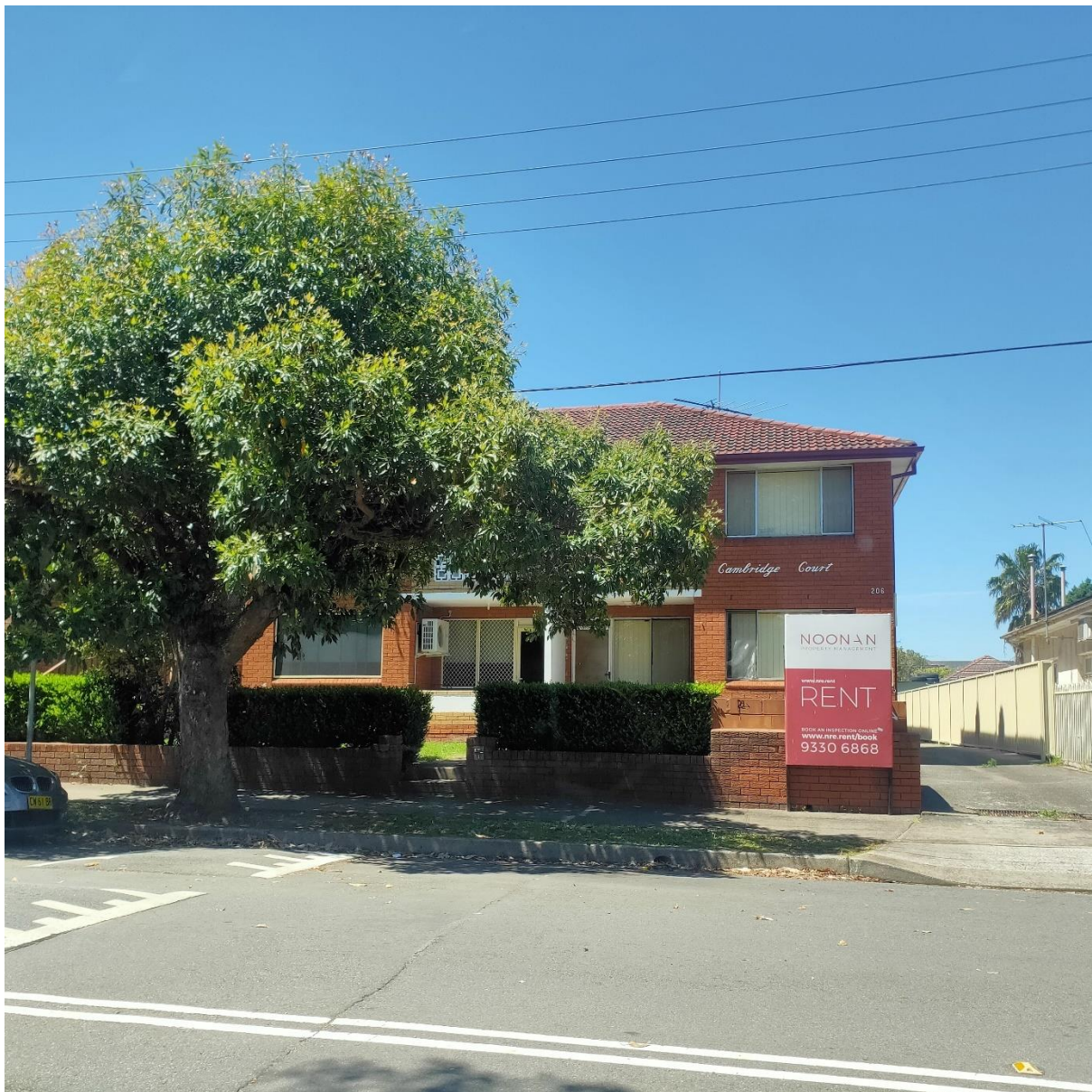
Fig.5 Photograph of adjoining two storey residential flat building at No. 204-206 Victoria Road, Punchbowl adjoining the site to the north (Source: Maximus Developments Australia, 2023).
